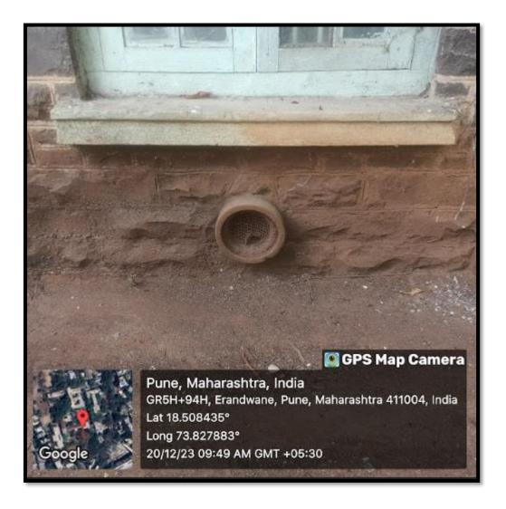
Due to the specific slope of the college building, a meticulous plan was devised to facilitate the drainage of percolating water away from beneath the structure, particularly during the monsoon season. This consideration was taken into account during the construction of the building at that time.
